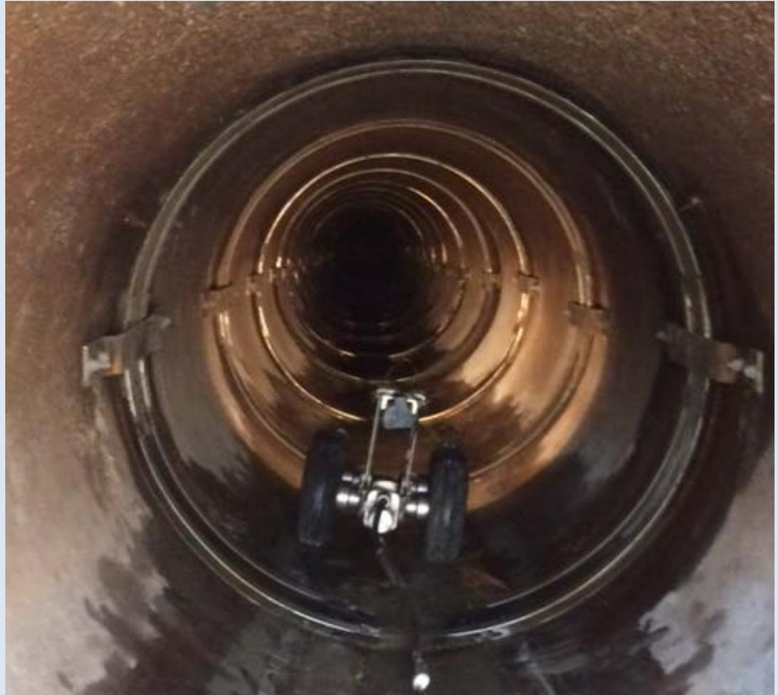
Joint Repair with Internal Bands and heavy-duty pipe ties.
