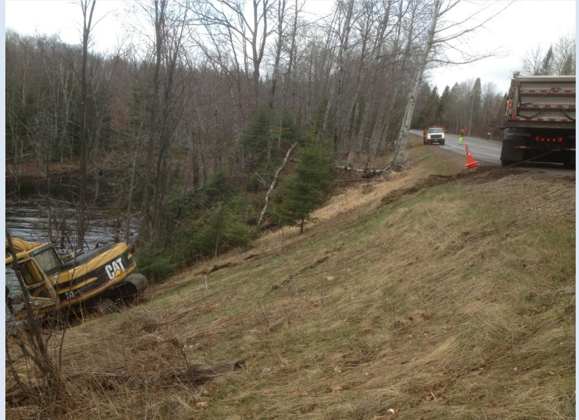
Beaver dam at RP 318.8 RT on TH 23. The box culvert is about 8' and the dam was about 7.5'. Not the best spot for the excavator to work in. We used tree about 14 inch in diameter and 25 feet long to break it loose.
